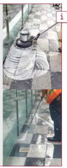
After jointing, in order to more or less remove the resulting synthetic resin film, clean the stone surface **immediately after sweeping** using a 1:20 ROMPOX® - BA-SIC CLEANING AGENT EXTRA: water mix by wiping over several times.
